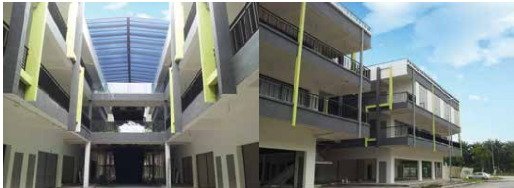
90% completed – actual site photo taken on Dec 2013
